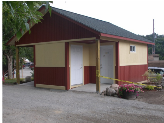
The new public accessible washrooms are finished and are looking great.
