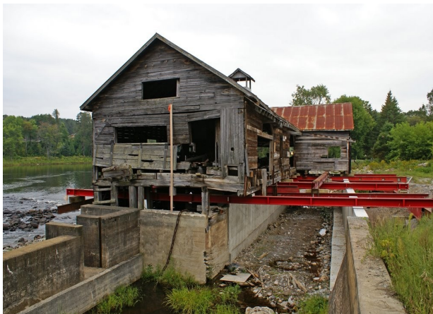
Clockwise from Top: The Mill Complex circa 1910 at its height of prosperity; the new viewing gallery is under construction; the red beams support the mill as the foundation goes in.
