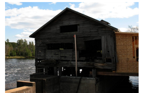
Clockwise from Top: The Mill Complex circa 1910 at its height of prosperity; the new viewing gallery is under construction; the red beams support the mill as the foundation goes in.
